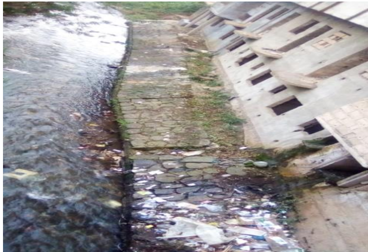
Figure 4: Construction site along Shut stream.
